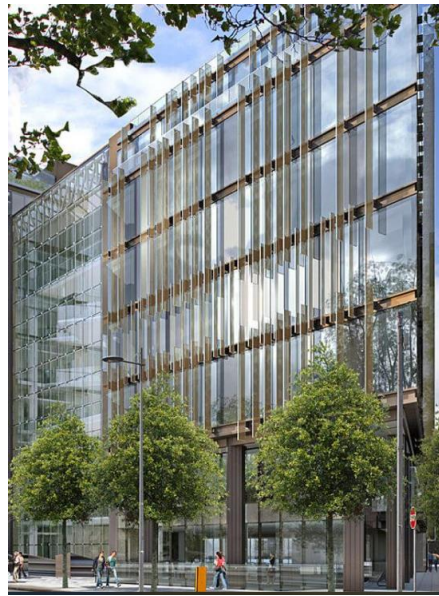
Figure 1. An example of a façade with large glass panes and external glass fins
